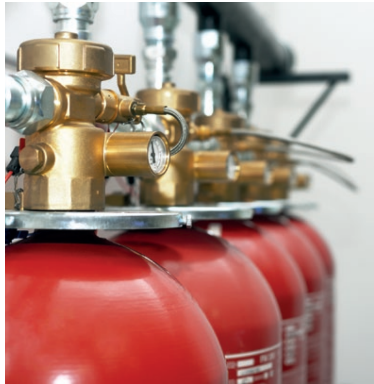
Extinguishing gas battery
