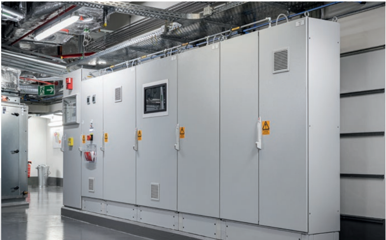
Switch cabinets protected with a nitrogen extinguishing system
