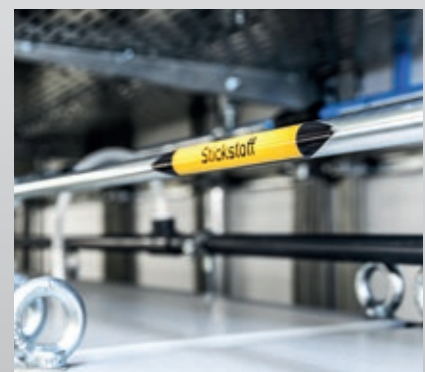
Nitrogen extinguishing line and suction pipe
